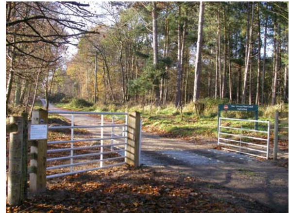
New gates and cattle grids have being installed to cater for access around the Forest. It is hoped that as the project area increases the fences will be relocated around any new project boundary.
